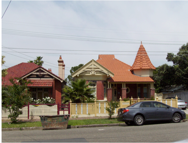
Figure 29.19 Challis Avenue. The candle snuffer roof is original, although re-tiled. It is the only such roof in the area and is rare in Marrickville.
